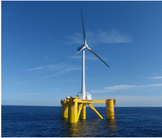
2MW Downwind-type Floating Wind Turbine “Fukushima Mirai” (Floater: 4 Column Semi-Sub)
